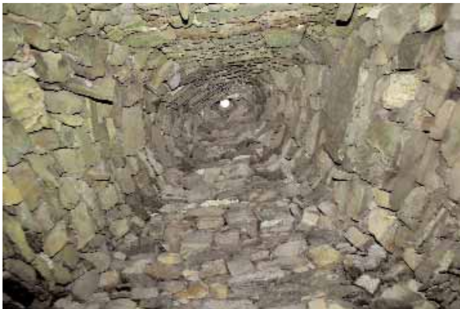
Pl. 32 - The inner dome of Cell F, showing corbelling and projecting stone pegs.
