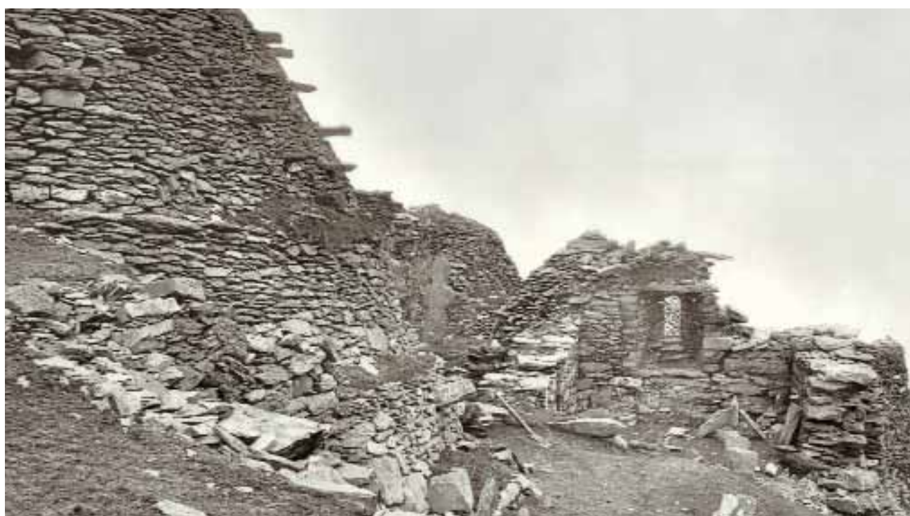
Pl. 7 - View of St Michael's Church, showing collapsed retaining wall on the south side, published in 'Notes on Irish Architecture'.
