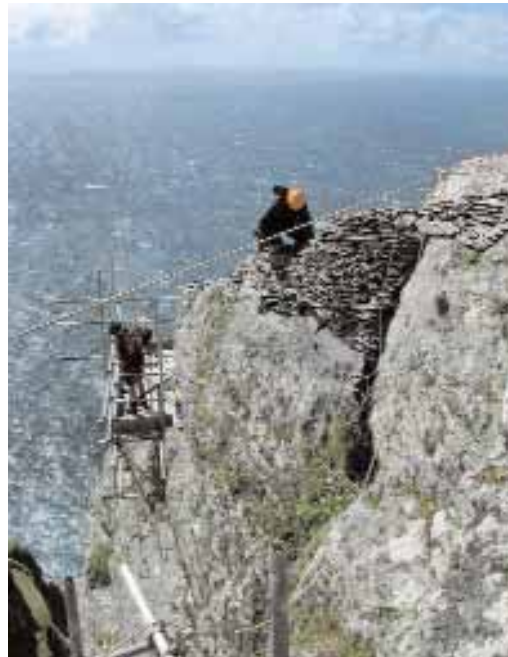
Pl. 14 - Working on the stabilisation of structures on the South Peak.
