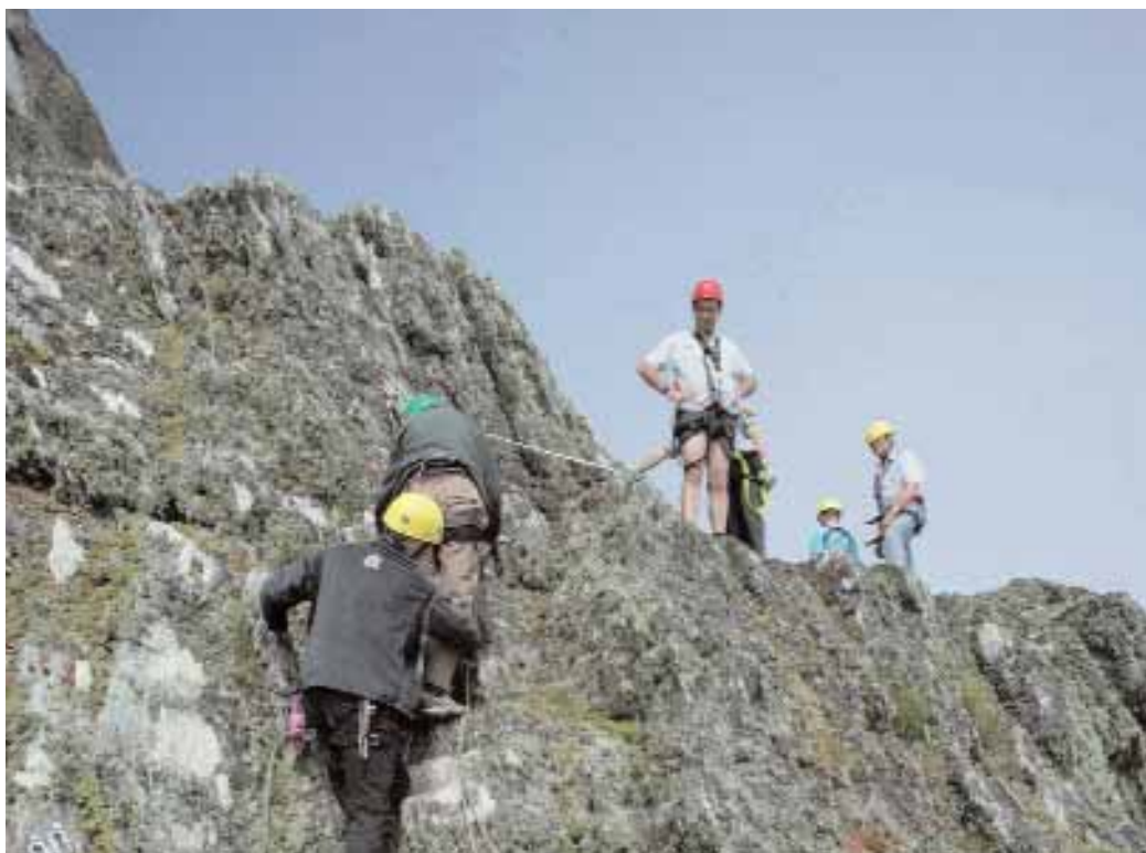
Pl. 15 - Working on the South Peak aided by ropes and overseen by a full-time Safety Officer.
