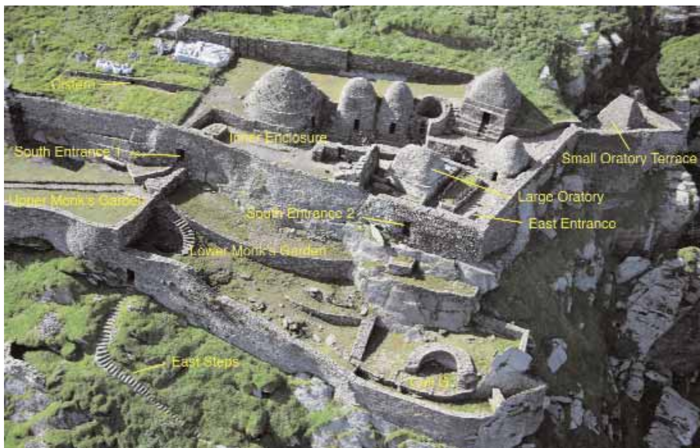
Pl. 4 - Aerial view of the Monastery, showing the inner enclosure (illustrating location of cells, oratories, church and leachta of the Lower Monks' Garden, with the remains of an earlier cell (G)). This view also shows top of the East Steps and original entrance into the Monastery.
