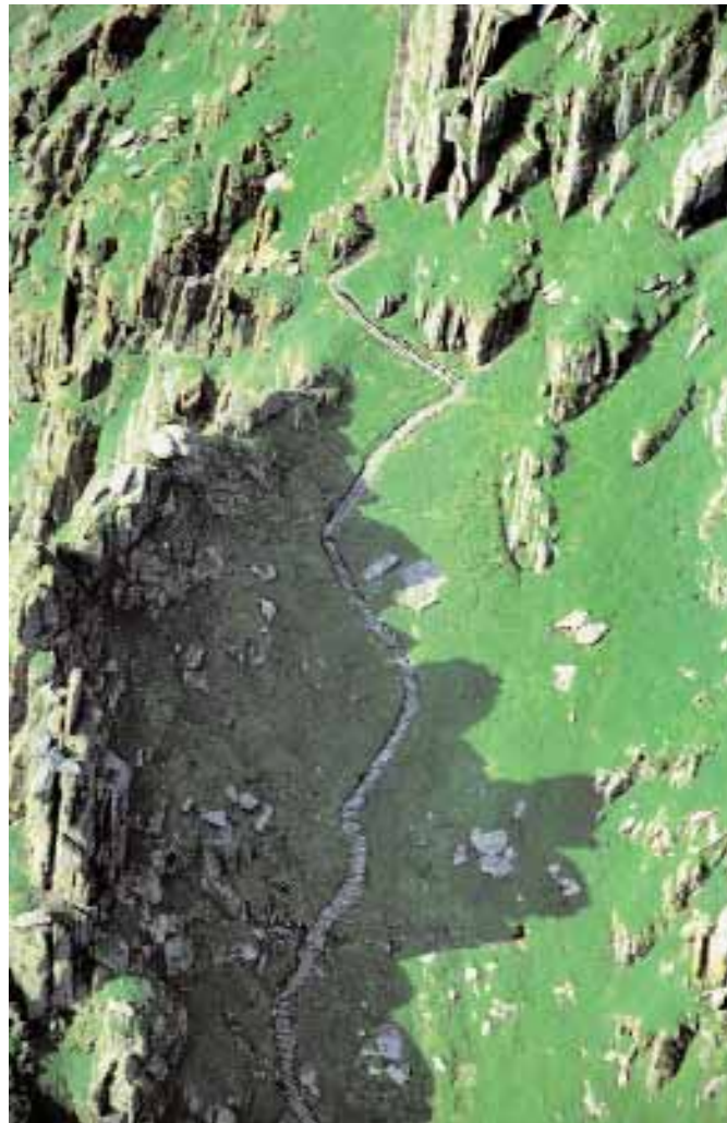
Pl. 24 - Aerial view of the East Steps.
